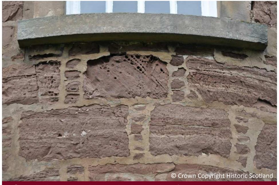
Classic 'honeycomb' weathering and surface loss caused by the action of salt spray and wind in a coastal location
