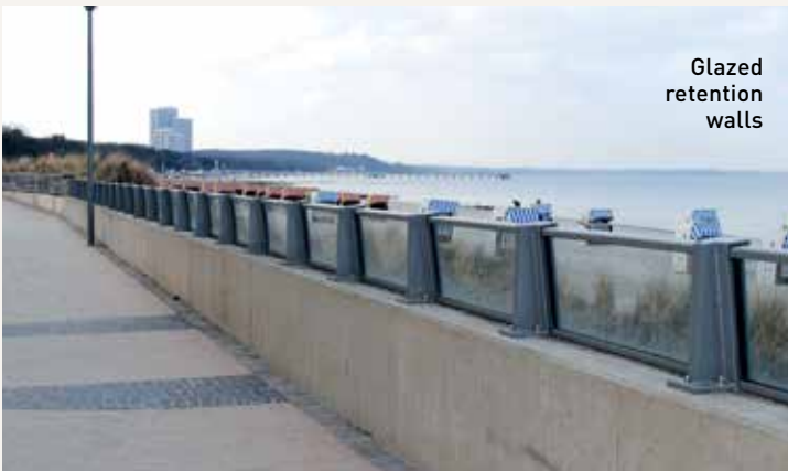
Construction of landscaping measures
