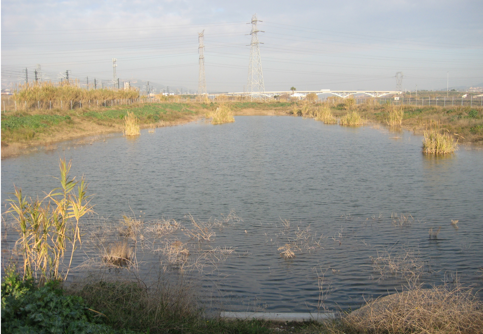
Copyright: Cetaqua Caption: MAR infiltration system in Sant Vicenç dels Horts (Barcelona, Spain).
