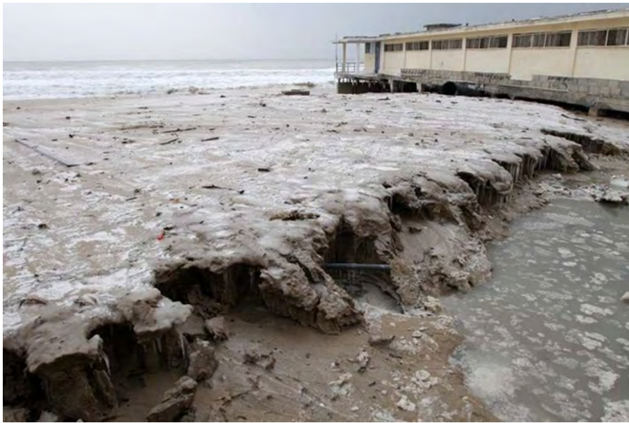
Figure 2.9 Flooding of Varna Central beach (north), undermining of Sea Baths foundation, damages to the buildings and beach erosion (Source: dariknews.bg).
