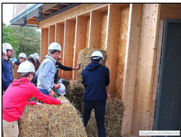
Figure 2 Installation of straw panels as building insulation
