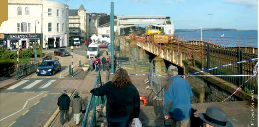
A view on Dawlish train station after the February 2014 storm
